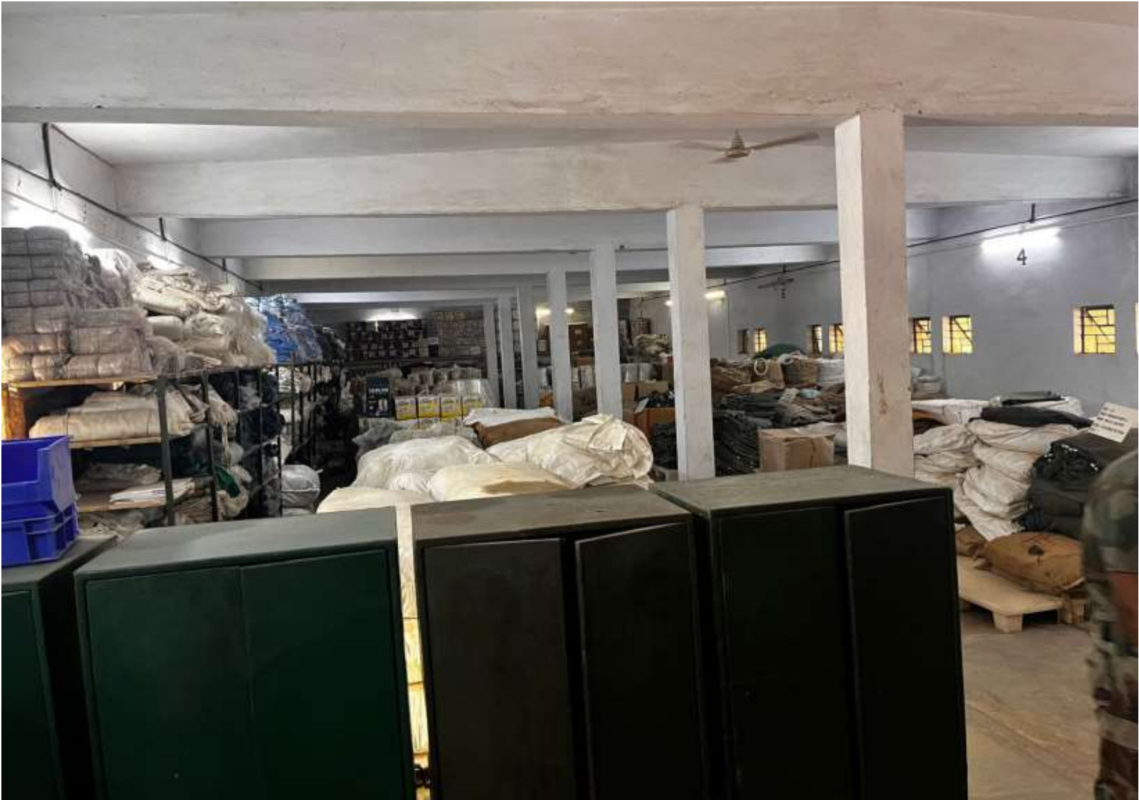
Existing Shed - Clothing Shed (Before)
