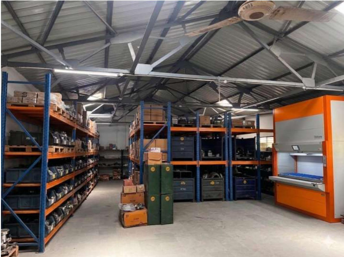
Existing Shed - MT Store (After)
