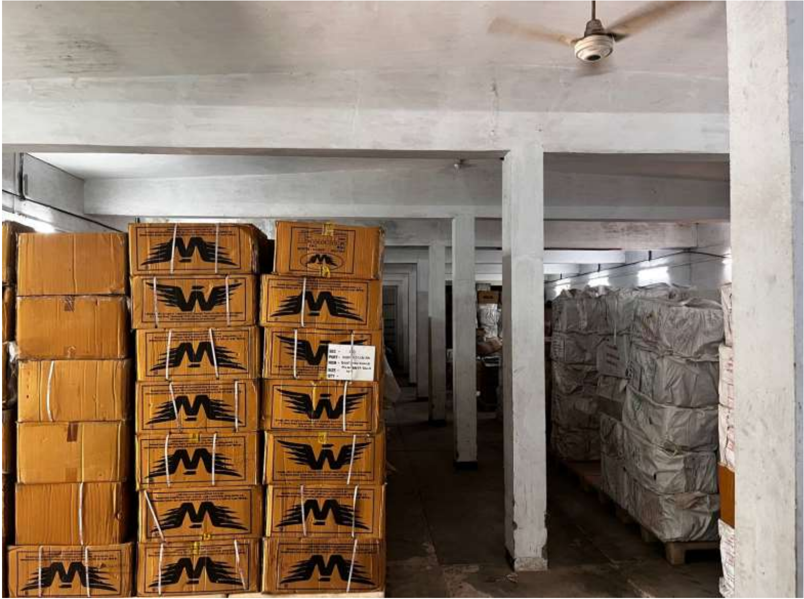
Existing Shed – Shed 3 (Before)
